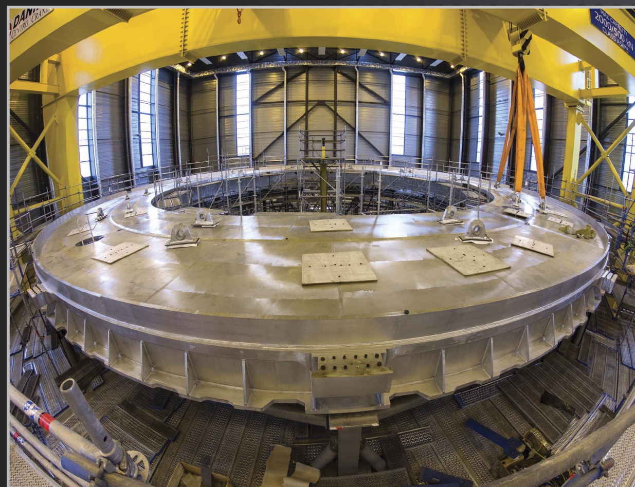
The assembly of the ITER cryostat is progressing under the responsibility of the Indian Domestic Agency, whose scope includes the fabrication, assembly, welding and testing of the four major cryostat sections, as well as final in-pit installation and welding.
